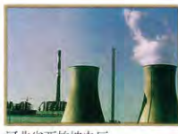
河北省西柏坡电厂 Hebei Power Station
