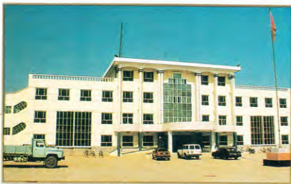
总公司办公楼 Office Building of the Corporation
